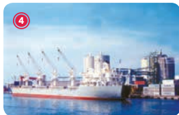
4 TERMINAL TANJUNG PRIOK Jakarta, DKI Jakarta
